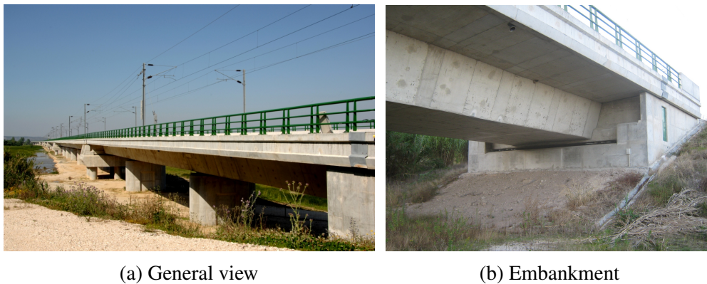
Figure 1: Santana do Cartaxo viaduct
