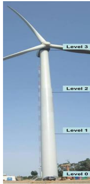
Figure 1 - Instrumented tower and levels position.
