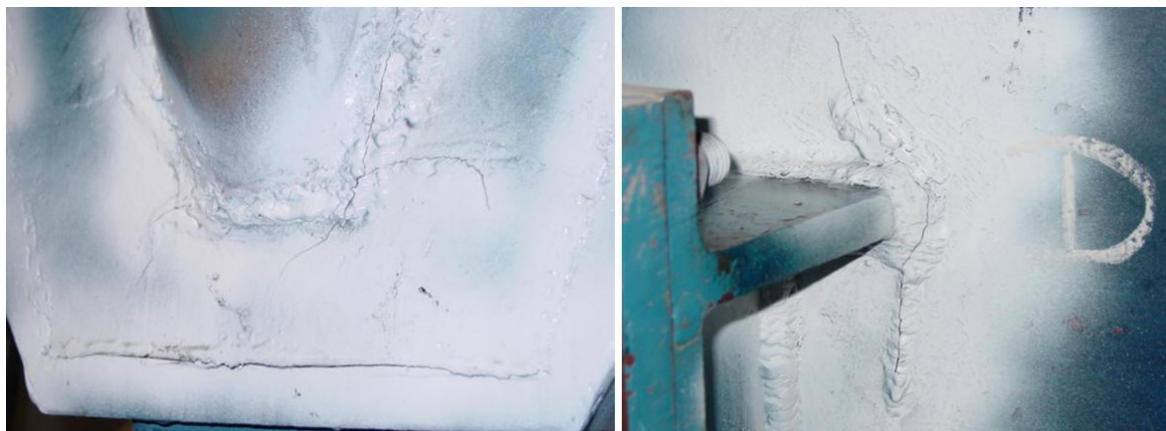
Figure 6: Example of cracks of the steel structure of the roller mill.
