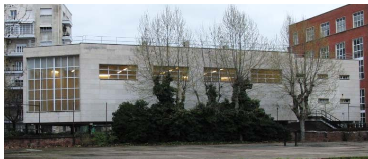
Figure 1: External photograph of the structure
