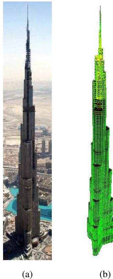
Figure 1: Burj Khalifa Bin Zayid : (a) building completed in 2009 in Dubai, United Arab Emirates and (b) corresponding numerical model in finite element.
