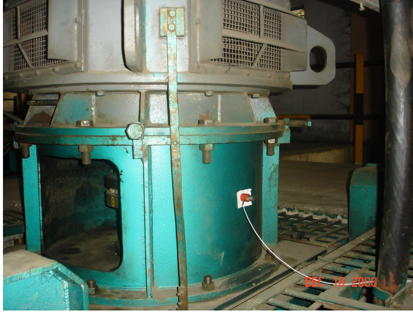
Figure 3 View of accelerometer placed on the motor stool.
